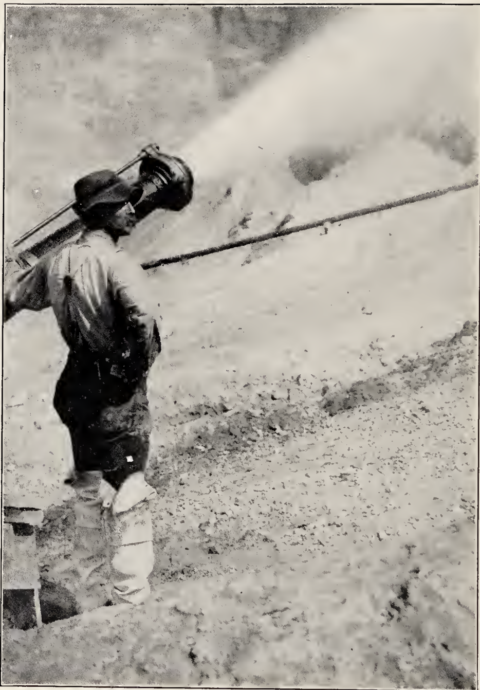
With all the force of a shell from a big gun, a giant stream of water is played against the hillside, washing the earth into sluice boxes, where a layer of mercury catches even the most infinitesimal particles of gold.
